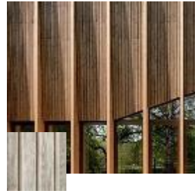
TIMBER CLADDING Preferred: Thermowood or similar
