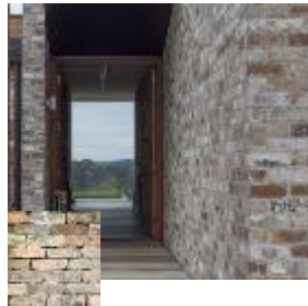
BRICK Preferred: reclaimed and assembled with lime mortar to absorb CO 2 .
